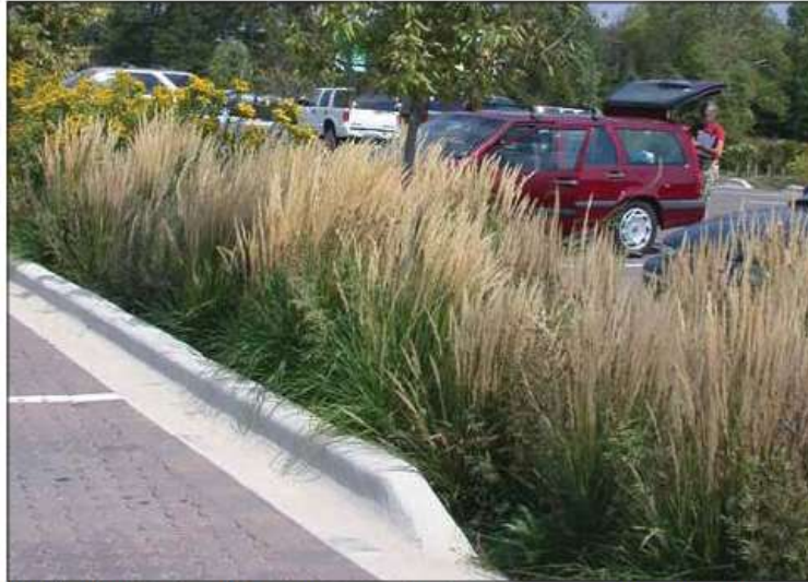
Parking lot islands and permeable paving for stormwater management
