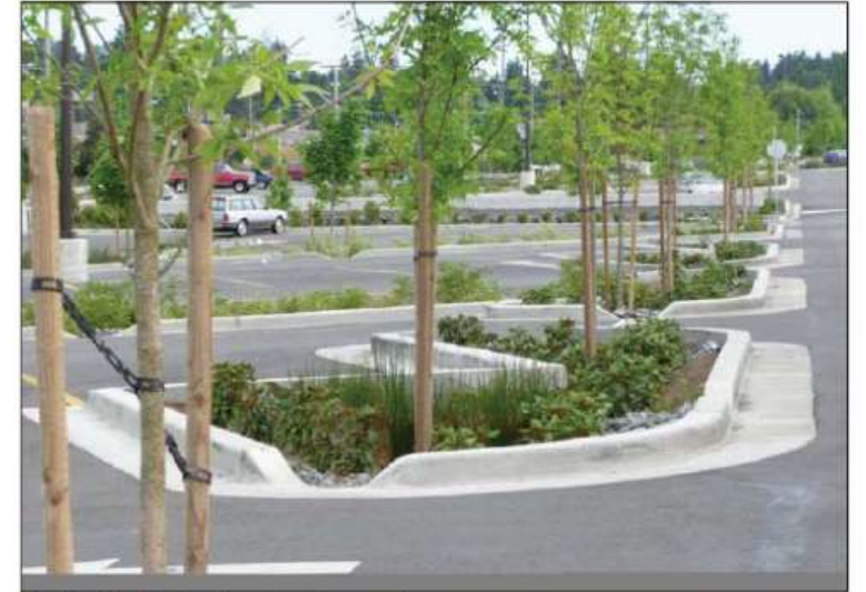
Parking lot bio-infiltration planters for stormwater management
