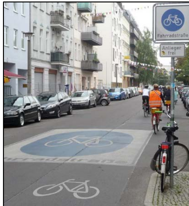
Figure 15: Slow Street Slow streets are designed for very low speed use by giving pedestrians and bicyclists priority while limiting motor vehicle speeds. Slow streets are known by a variety of names including play streets, low speed streets, and “woonerfs” after their Dutch name. The streets are generally at sidewalk level, without curbs. Motor vehicles are allowed to use the street to gain access to homes, businesses, or parking, but at very low speeds. Often the street is designed with chicanes or street furniture that forces vehicles to meander and move at a very slow pace. Many European countries have turned other lower volume residential streets into slower streets using a variety of treatments.
