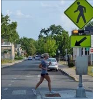
Figure 20: Rectangular Rapid Flashing Beacons (RRFBs)
