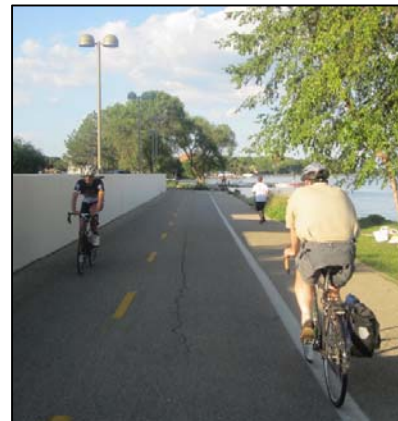
Figure 35: Shared-Use Path A shared use path is an off-street bicycle and pedestrian facility that is physically separated from motor vehicle traffic. Typically shared use paths are located in an independent right-of-way such as in a park, stream valley greenway, along a utility corridor, or an abandoned railroad corridor. Shared-use paths are used by other non-motorized users including pedestrians, skaters, wheelchair users, joggers, and sometimes equestrians.
