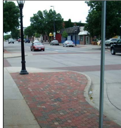
Figure 22: Pedestrian Bump-out / Curb Extension
