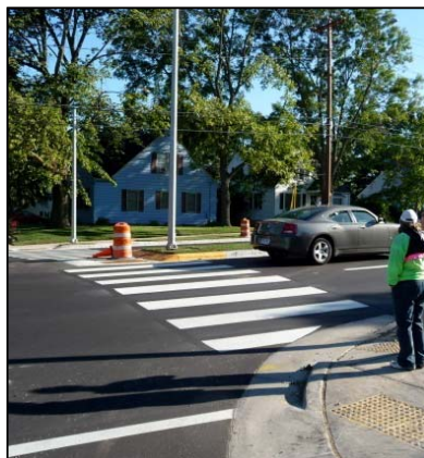
Figure 17: Crosswalk: Marked Marked crosswalks emphasize and designate the part of an intersection where drivers can expect pedestrians to cross. They also define the pedestrian crossing area where they otherwise would not exist such as a mid-block crossing. Motorists must always yield the right of way to pedestrians in any crosswalk except at a signalized intersection where pedestrians follow the appropriate signal. Crosswalks may be marked with two parallel lines (“standard”) or with wide bars that run in the direction of traffic (“continental,” shown here). Continental crosswalks are more visible to motorists than standard crosswalks.
