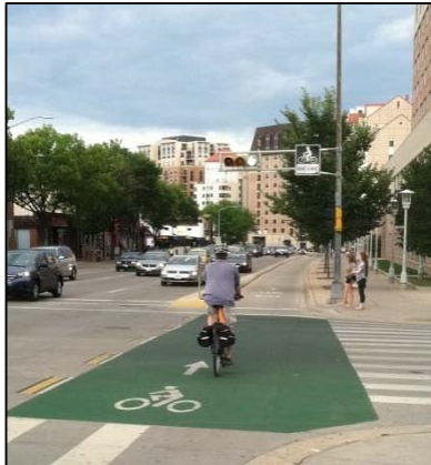
Figure 36: Colored Pavement Green colored pavement may be used to increase the visibility of bicycle facilities. Colored pavement may be used to highlight an entire bicycle corridor, but is most useful to highlight bicycle facilities in conflict areas – through intersections, across driveways, or crossing highway ramps.
