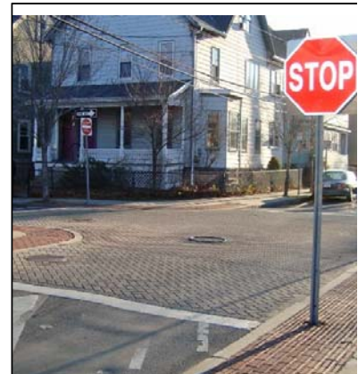
Figure 16: Raised Intersection Raised intersections elevate an entire intersection to the level of the curb and sidewalk, essentially creating a large speed table. Like raised crosswalks, raised intersections crosswalks encourage motorists to yield to pedestrians because the raised intersection increases pedestrian visibility and forces motorists to slow down before going over the speed table. The crosswalks on each approach to a raised intersection are also elevated to enable pedestrians to cross the road at the same level as the sidewalk, eliminating the need for curb ramps. Raised intersections may use standard paving materials such as concrete or asphalt, or may use materials such as brick or other pavers to further differentiate the space.
