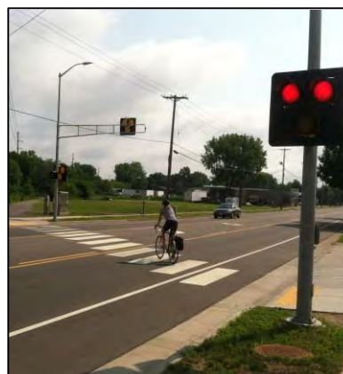
Figure 19: Pedestrian Hybrid Beacon ("HAWK") A pedestrian hybrid beacon is an overhead warning device, used at locations that are unusually hazardous or where pedestrians or bicyclists should be expected to cross throughout the day or where pedestrian crossing activity would not be readily apparent. The beacon is dark until activated by a pedestrian or bicyclist. When activated, the beacon displays a yellow signal followed by a red signal to drivers and a "walk" signal to pedestrians. Criteria for installation are available in the MUTCD.
