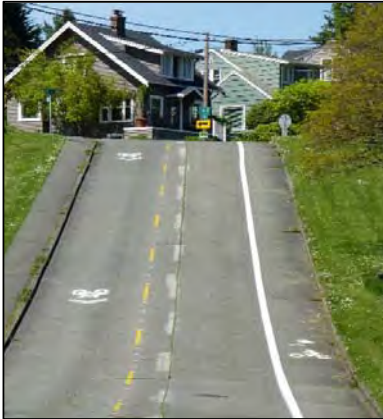
Figure 30: Bike Lane – Climbing A climbing lane provides a bicycle lane or buffered bicycle lane in the uphill direction on a hill, and shared lane markings in the downhill direction. This is often done where there is not room to fit a bicycle lane on each side of the street; providing a bicycle lane uphill allows slow moving bicyclists to move out of the travel lane. Bicyclists traveling downhill are often moving much closer to the speed of motor vehicles, and shared lane markings help position bicyclists in the most appropriate location to ride while also providing a visual cue to motorists that bicyclists have a right to use the street.
