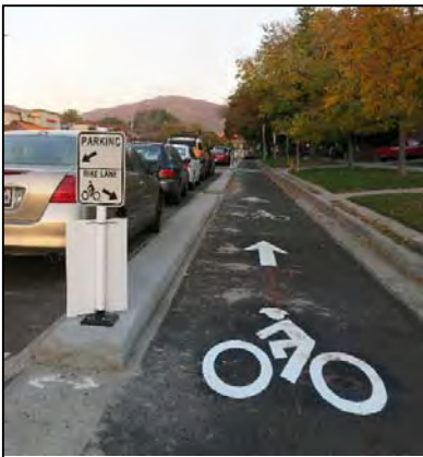
Figure 29: Bike Lane – Separated Separated bike lanes, sometimes called “cycle tracks” or “protected bike lanes,” separate the bike lane from travel lanes with a vertical element such as curbs, bollards, pavement elevation, parked cars, or planters. While separated bike lanes increase bicyclists’ sense of comfort, they still have conflict points at intersections and driveways, where turning traffic crosses them. Separated bike lanes may be placed at street level, sidewalk level, or an intermediate level, and may include vertical or rolled curbs. Preferred Width: 6.5 feet plus gutter pan (one way); 10+ feet plus gutter pan (two-way) Minimum Width: 5 feet plus gutter pan (one-way); 8 feet plus gutter pan (two-way)
