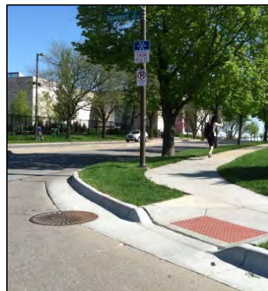
Figure 18: Crosswalk: Unmarked In Wisconsin, unmarked crosswalks are the continuation from a sidewalk on one side of the street to the other side of the street. Motorist must always yield the right of way to pedestrians in any unmarked or marked crosswalk except at a signalized intersection where pedestrians follow the appropriate signal.
