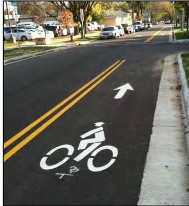
Figure 31: Bike Lane – Contraflow Counter-flow bike lanes are signed and marked lanes that accommodate bicycle travel on one-way streets in the opposite direction of motor vehicle traffic. Counter-flow bike lanes may be conventional bike lanes, buffered bike lanes, or fully separated bike lanes.
