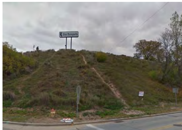
Figure 45: Existing Conditions – Location of Proposed Staircase
