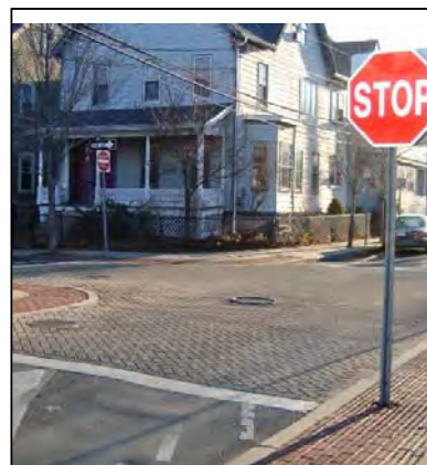
Figure 16: Raised Intersection Raised intersections elevate an entire intersection to the level of the curb and sidewalk, essentially creating a large speed table. Like raised crosswalks, raised intersections crosswalks encourage motorists to yield to pedestrians because the raised intersection increases pedestrian visibility and forces motorists to slow down before going over the speed table. The crosswalks on each approach to a raised intersection are also elevated to enable pedestrians to cross the road at the same level as the sidewalk, eliminating the need for curb ramps. Raised intersections may use standard paving materials such as concrete or asphalt, or may use materials such as brick or other pavers to further differentiate the space.
