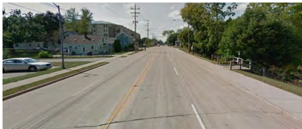
Figure 48: Packard Street – Existing Conditions
