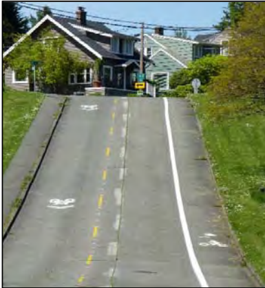
Figure 30: Bike Lane – Climbing A climbing lane provides a bicycle lane or buffered bicycle lane in the uphill direction on a hill, and shared lane markings in the downhill direction. This is often done where there is not room to fit a bicycle lane on each side of the street; providing a bicycle lane uphill allows slow moving bicyclists to move out of the travel lane. Bicyclists traveling downhill are often moving much closer to the speed of motor vehicles, and shared lane markings help position bicyclists in the most appropriate location to ride while also providing a visual cue to motorists that bicyclists have a right to use the street.
