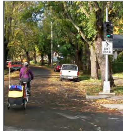
Figure 38: Bike Signal Bicycle signals are traffic signals that govern bicycle movements at an intersection. Bicycle signals may be used when bicycles, pedestrians, and motor vehicles have different movement cycles.
