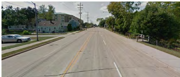
Figure 48: Packard Street – Existing Conditions
