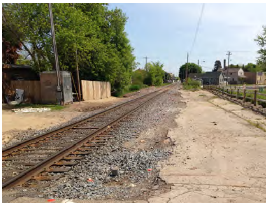
Railroad tracks represent infrastructure barriers and require specific improvements for a safe crossing along bike and pedestrian routes. They also provide opportunities for parallel routes.
