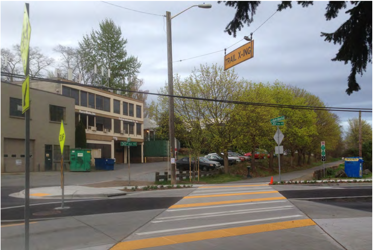
High visibility crossings and clear signage create continuity in the trail system at intersections with roadways.
