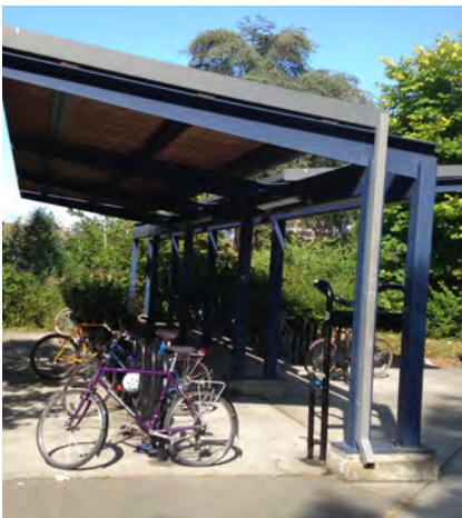
Covered bicycle parking provides protection from inclement weather for short term parking. A bike repair station is also located under the shelter in the example to the left.
