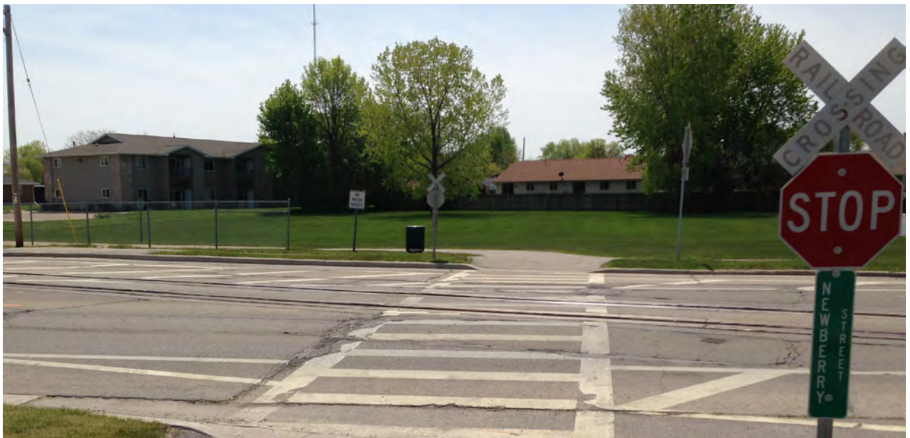
Upgrade projects, such as improved crossings with roadways and rail lines, can improve trail safety and increase comfort a wide range of trail users.
