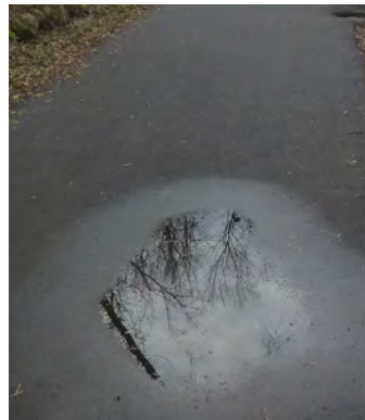
Sags: Specific depressions of pavement due to settlement or displacement due to tree roots
