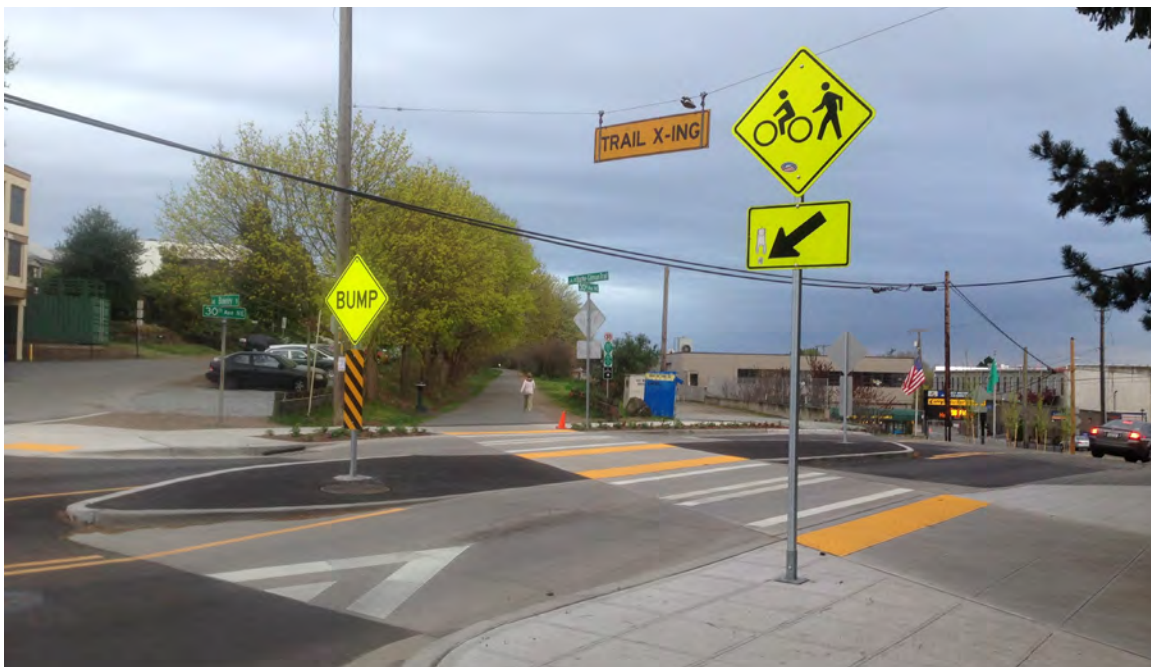
This raised crosswalk on the Burke Gilman Trail in Seattle, WA includes features such as clear signage, detectable warning strips, and pavement markings to provide warning to trail users and vehicles that they are approaching an intersection.
