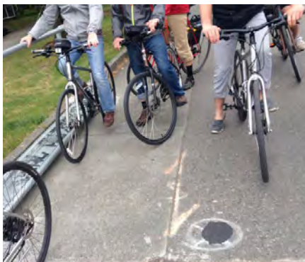
Radar Sensors (Source: Twitter user Dongho Chang, Traffic Engineer, Seattle Department of Transportation)
