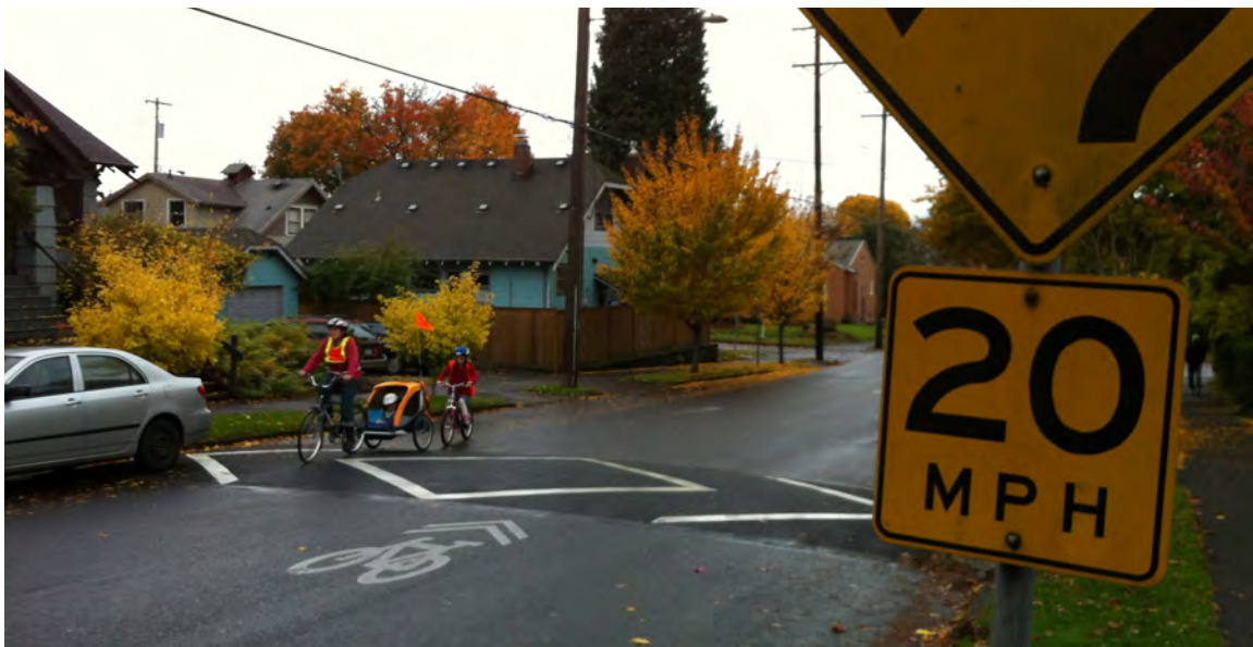
Speed and volume controls, including signs, pavement markings, and speed humps are used in this neighborhood bicycle boulevard in Portland, OR.
