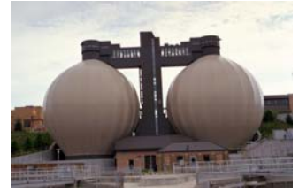
AWWTP egg-shaped anaerobic digesters.
