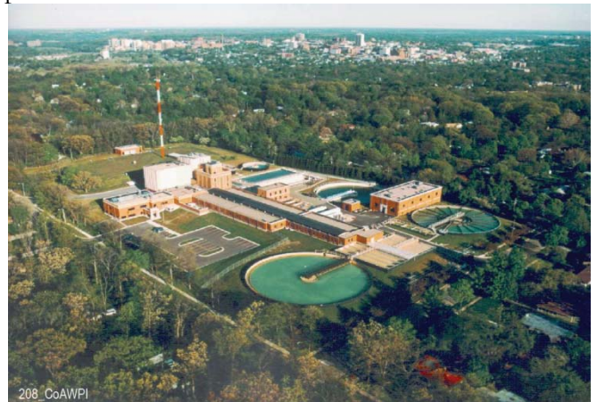
Ann Arbor Water Plant
