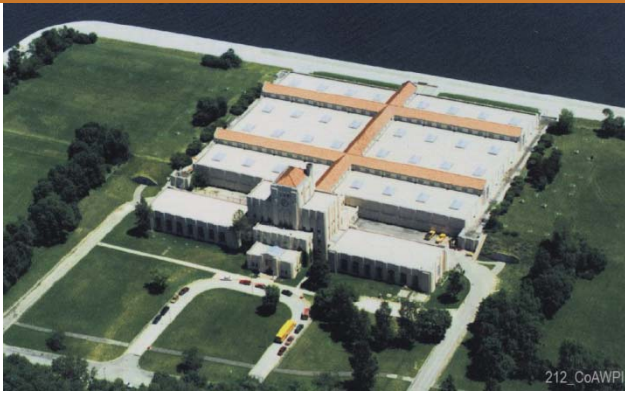
Linnwood Water Plant: 275 mgd
