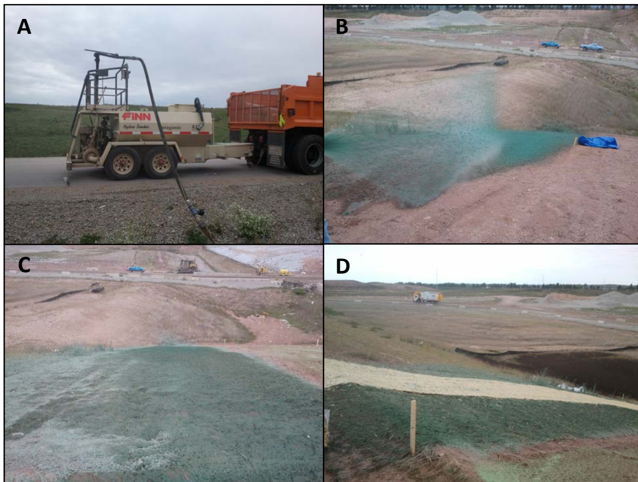
Figure 3.5: Preparation of plot six. A) Hydro seeder was used to apply the hydro mulch product (DS-150) B) Spraying of product onto plot C) Final application of hydro mulch D) Application of final straw matting
