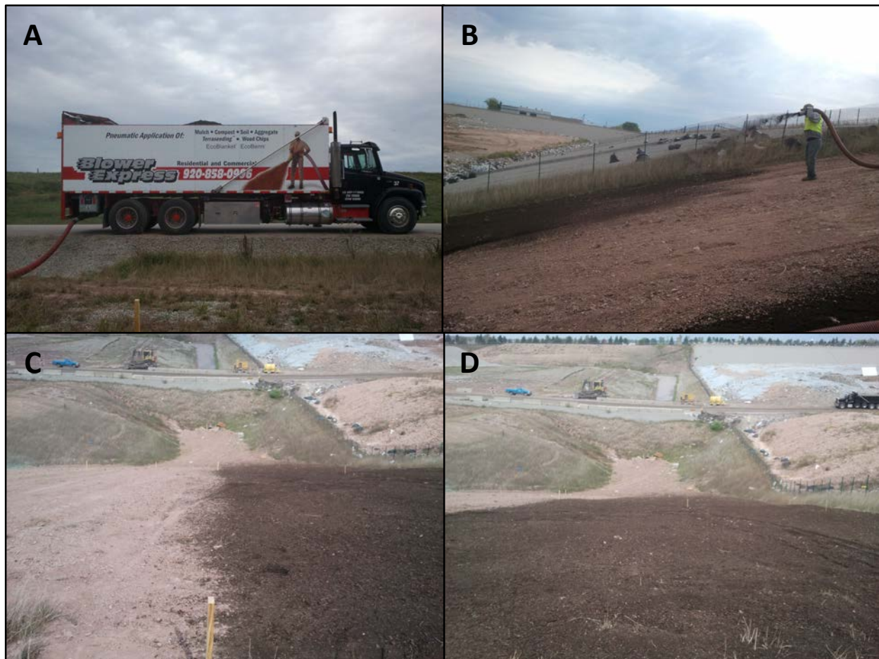
Figure 3.3: Preparation of plot one and two. A) Pneumatic blower truck used for application of compost material B) Application of blown compost C) View between plots two and three D) View of plots one and two after application of blown compost
