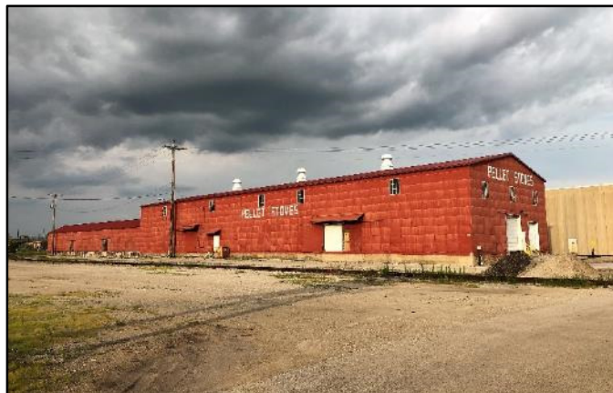
Fort Howard Lumber Company Warehouse, 1890 1095 S. Broadway, Green Bay
