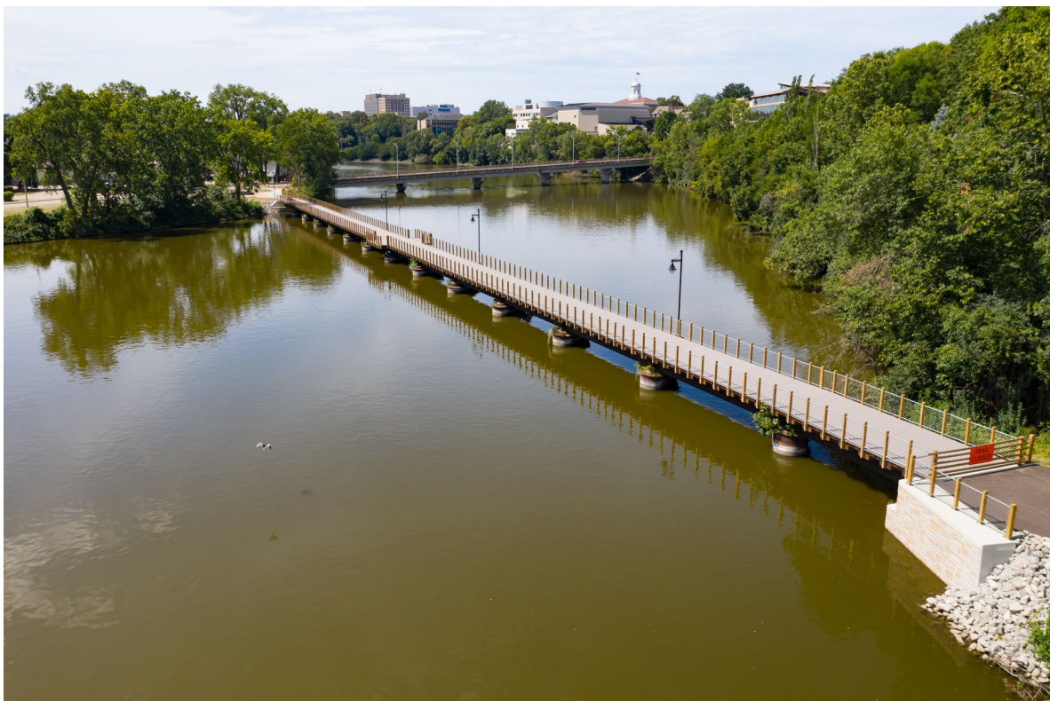
Lawe Street Trestle Conversion - 2020
