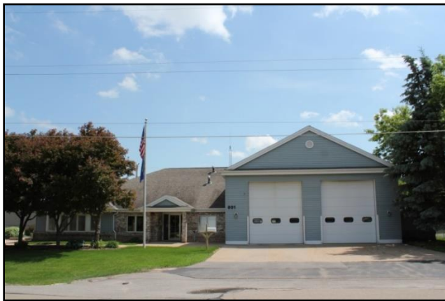
Fire Station #3 – 801 W. Grove Street
