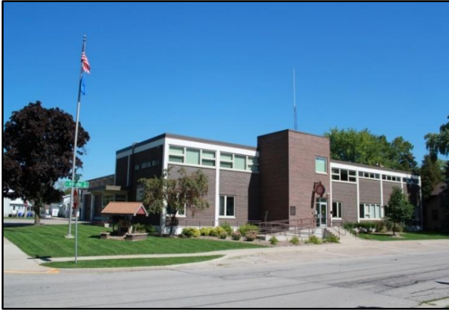
Fire Station #1 – 700 N. Drew Street
