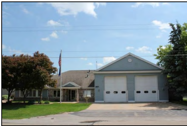
Fire Station #3 – 801 W. Grove ST
