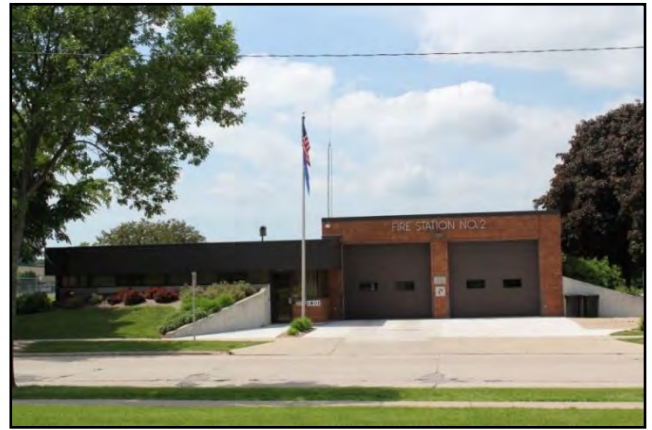
Fire Station #2 – 1801 S. Matthias ST
