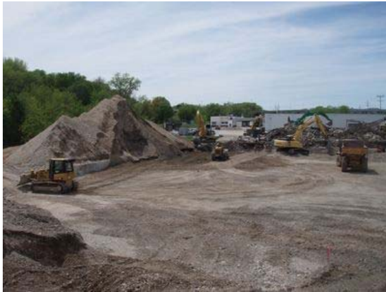
Ground breaking and site preparation
