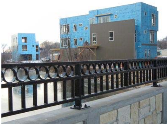
Nearly completed townhome unit
