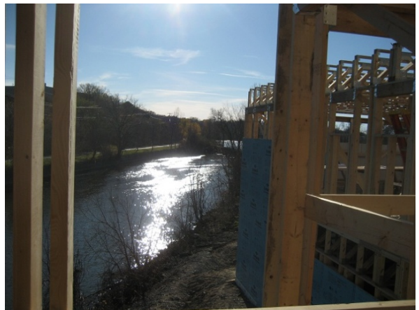
Townhome unit under construction
