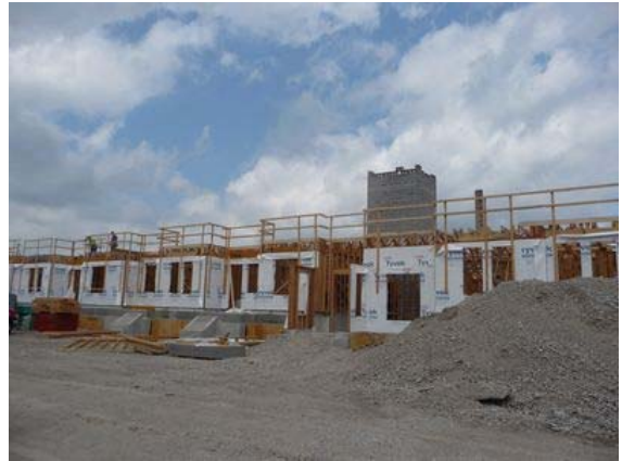
Eagle Flats under construction
