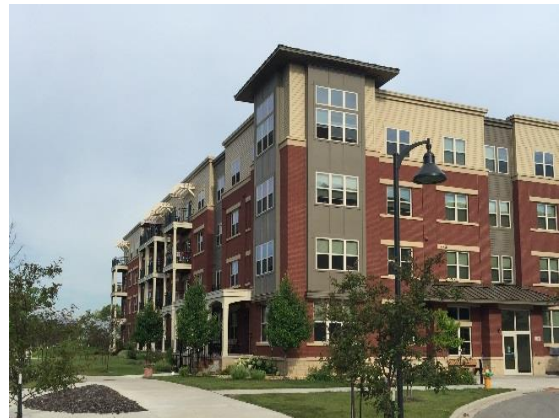
Riverwalk Place provides affordable senior housing
