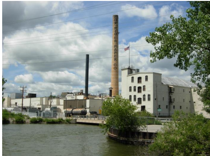
The mill race passes under the portion of Fox River Paper's building at far right, which may be considered for preservation along with the smokestack.
