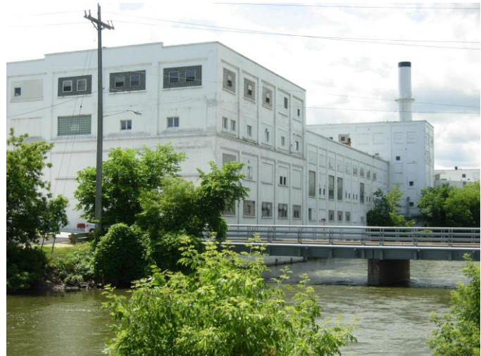
Riverside Paper's building abutting Lawe Street
