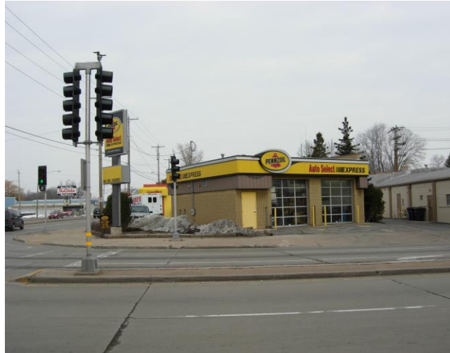
Northeast corner of Wisconsin Avenue and Richmond Street
