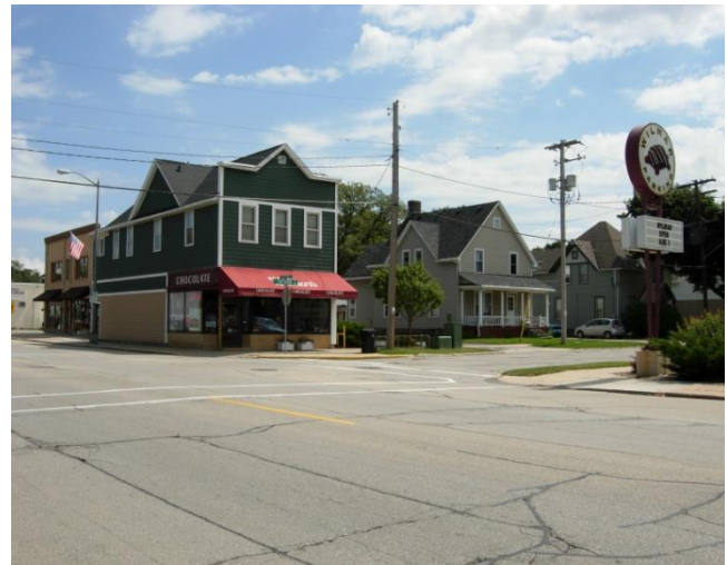
A remodeled building on Wisconsin Avenue
