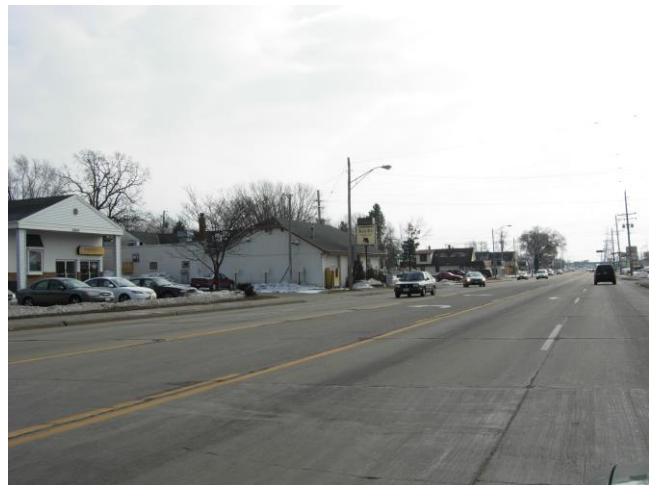
Typical conditions on South Oneida Street.
