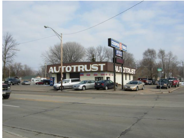
Example of a building that does not meet the City's standards for new construction.
