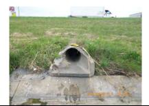
One side of the concrete apron is chipped.
