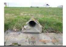
One side of the concrete apron is chipped.
