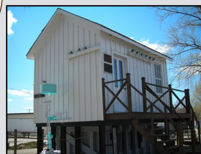
Vulcan Street Plant Replica
